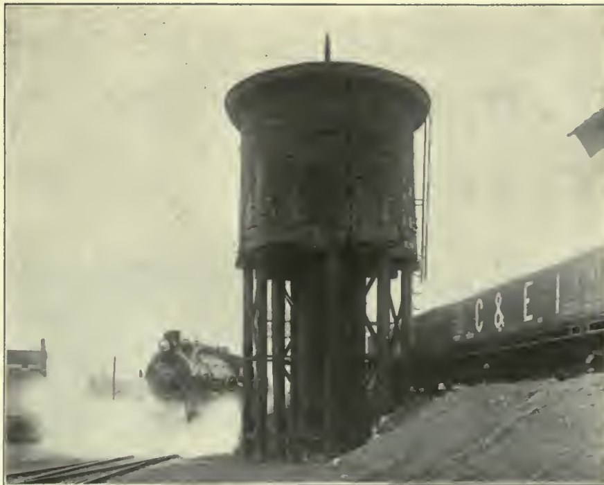
FIG. 660. FACILITIES TO BE ABANDONED. Wooden water tank of the Chicago, Rock Island & Pacific Railway, near 47th Street and Armour Avenue. This tank represents a type of railroad structure which is common in the city of Chicago. It has a capacity of about 35,000 gallons, and is a wooden tub on a wooden frame. In the event of electrification, tanks of this type will be rendered worthless in their present locations.
